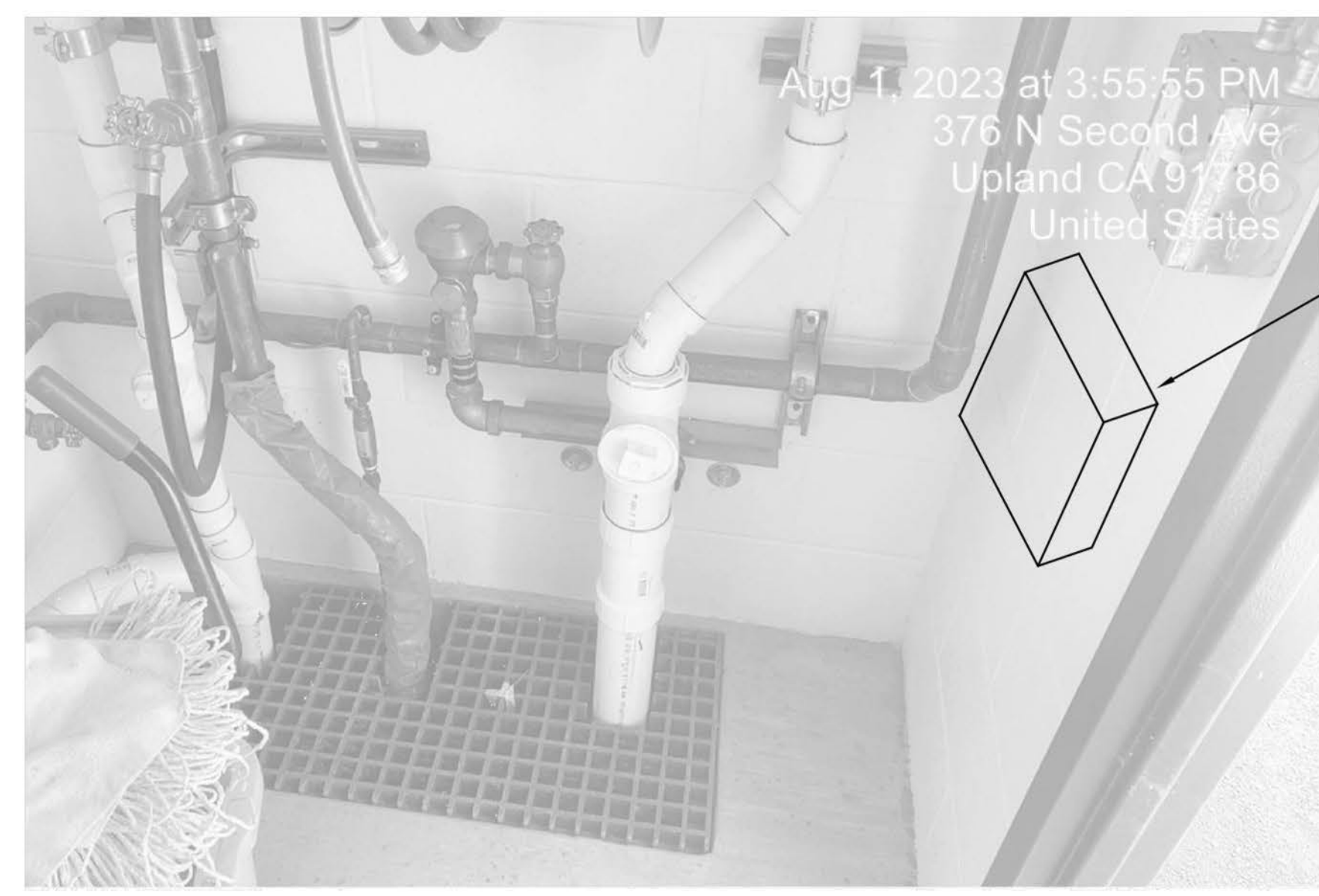
NORTHWEST CORNER OF EXISTING RESTROOM BUILDING
